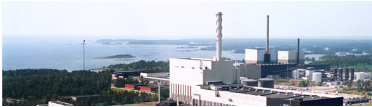
Figure 6 Picture of OKG's three reactors. Geographical position of OKG is on the Swedish east coast, 30 km north of Oskarshamn (OKG 1).
