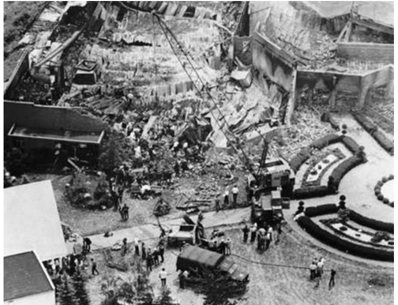
An aerial view of the fire scene.
