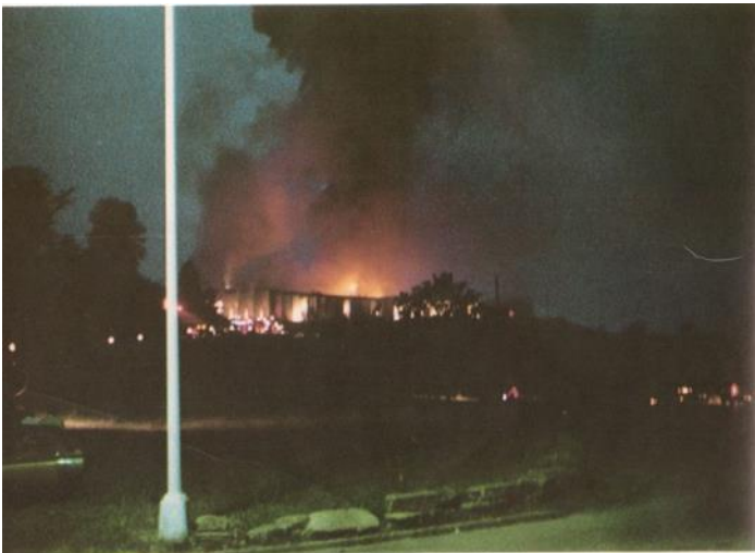
This is about 10:30, and the fire has spread throughout the building. One hour later, the building was on the verge of collapse, and the firemen were ordered out of the building.
