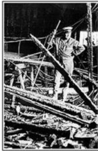
Aftermath: Debris from the 1970 fire. QZOOM
