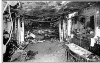
Lobby destroyed: The plush lobby where patrons enjoyed cocktails at the bar was reduced to a mass of tangled wiring and charred timbers. QZ00M
