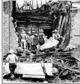
Searching for causes: Firefighters search remains of the Zebra Room with state investigators several days after most of it was incinerated. A room for small occasions, its paper-veneered paneling looked like shiny rosewood. Investigators determined that the room became a furnace when flashover (simultaneous ignition of all combustible materials) occurred. QZ00M
