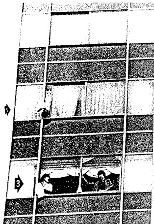
View of guests at windows shows variety of window conditions. (1) Window open to stop was extent of operation without removing stop. (2) Window open to stop, glass removed. (3) Window closed and two glass lights broken. (Credit: Las Vegas SUN)
