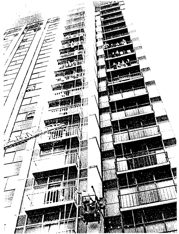
View of north face of hotel shows aerial ladder and construction hoist used to rescue some occupants. All but lowest (5th floor) guest room floors are shown. (Credit: Las Vegas SUN)
